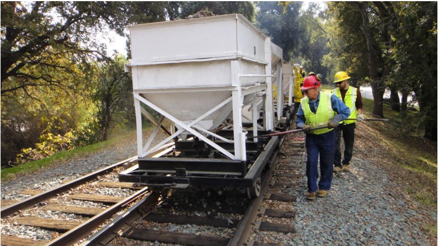
Clem and Chris M. disgorge the ballast rock between the rails filling in holes and low spots
