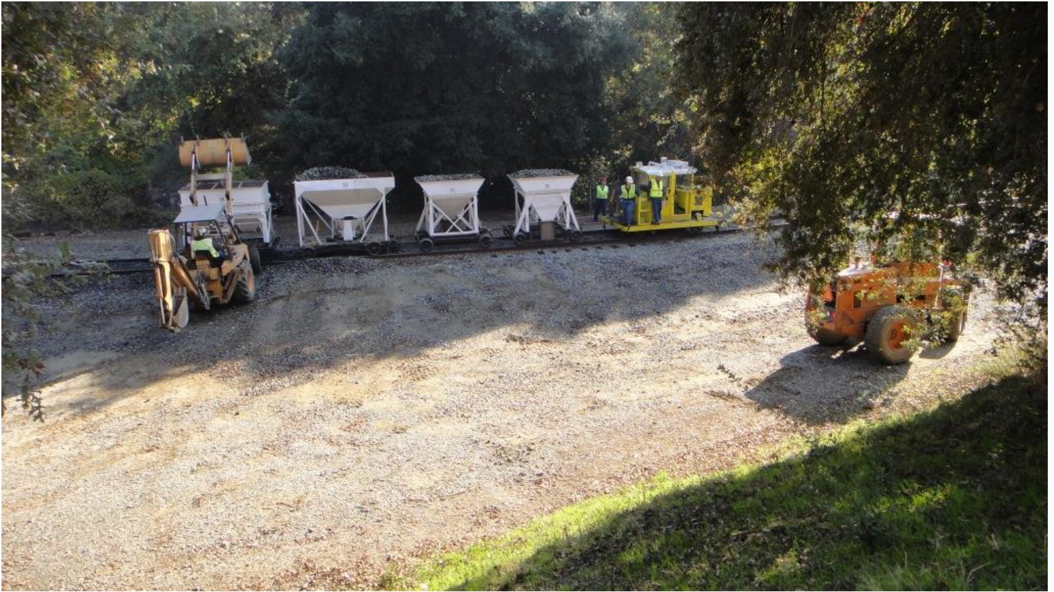
Frank in the back-hoe and Steve N. in the front-end loader fill the hoppers with rock
