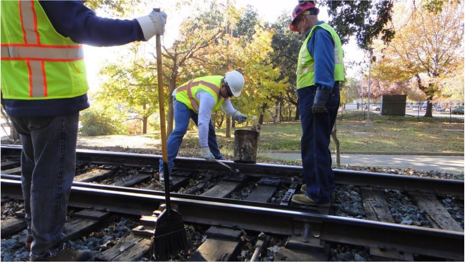
Initiation of the new guys! Chris N. gets his hands on the switch-grease bucket as Clem supervises
