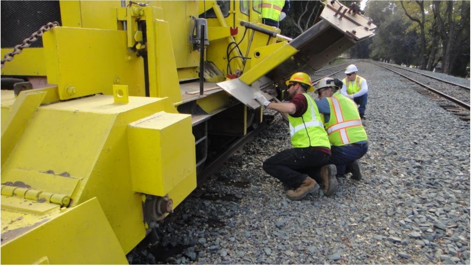
Chris M. and Alan work on making adjustments on the ballast regulator's wing to pull rock in towards the rail
