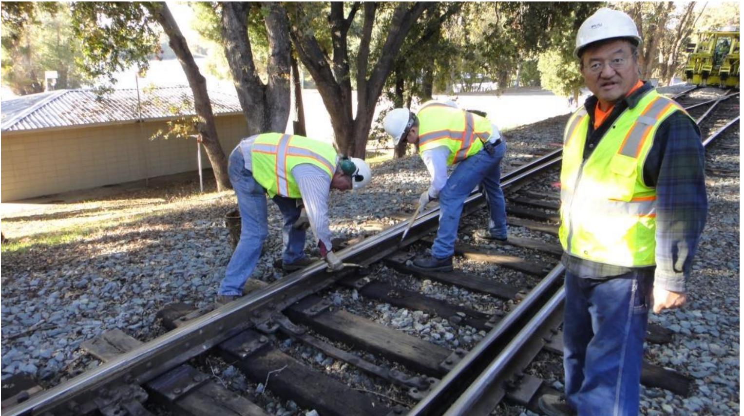
Team veteran Steve N. takes the grease brush as rookie Chris N. scrape old grease off switch-plates. John provides the color commentary
