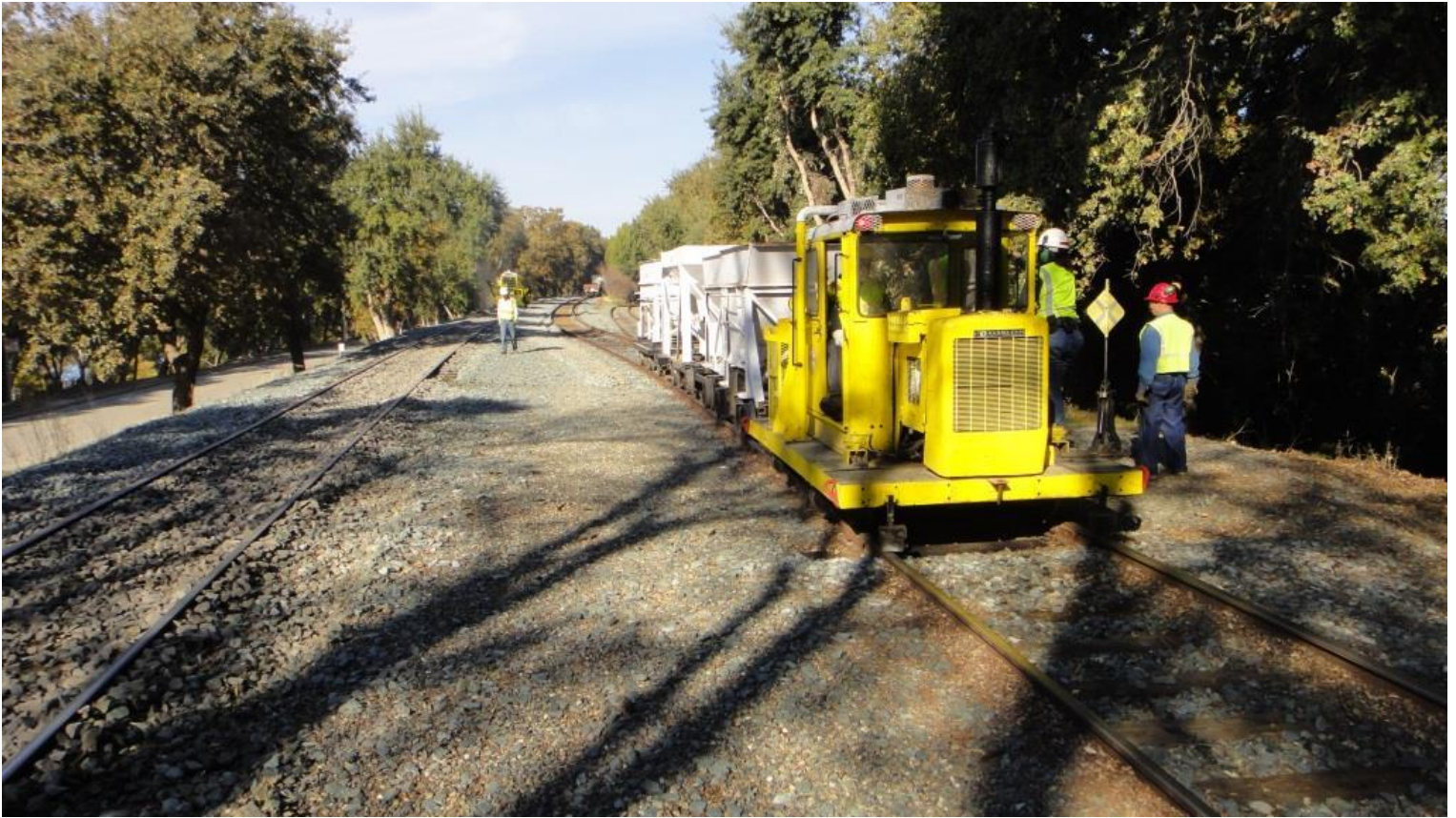
Team Tug prepare to run-around the ballast hoppers in preparation for pulling them back to town
