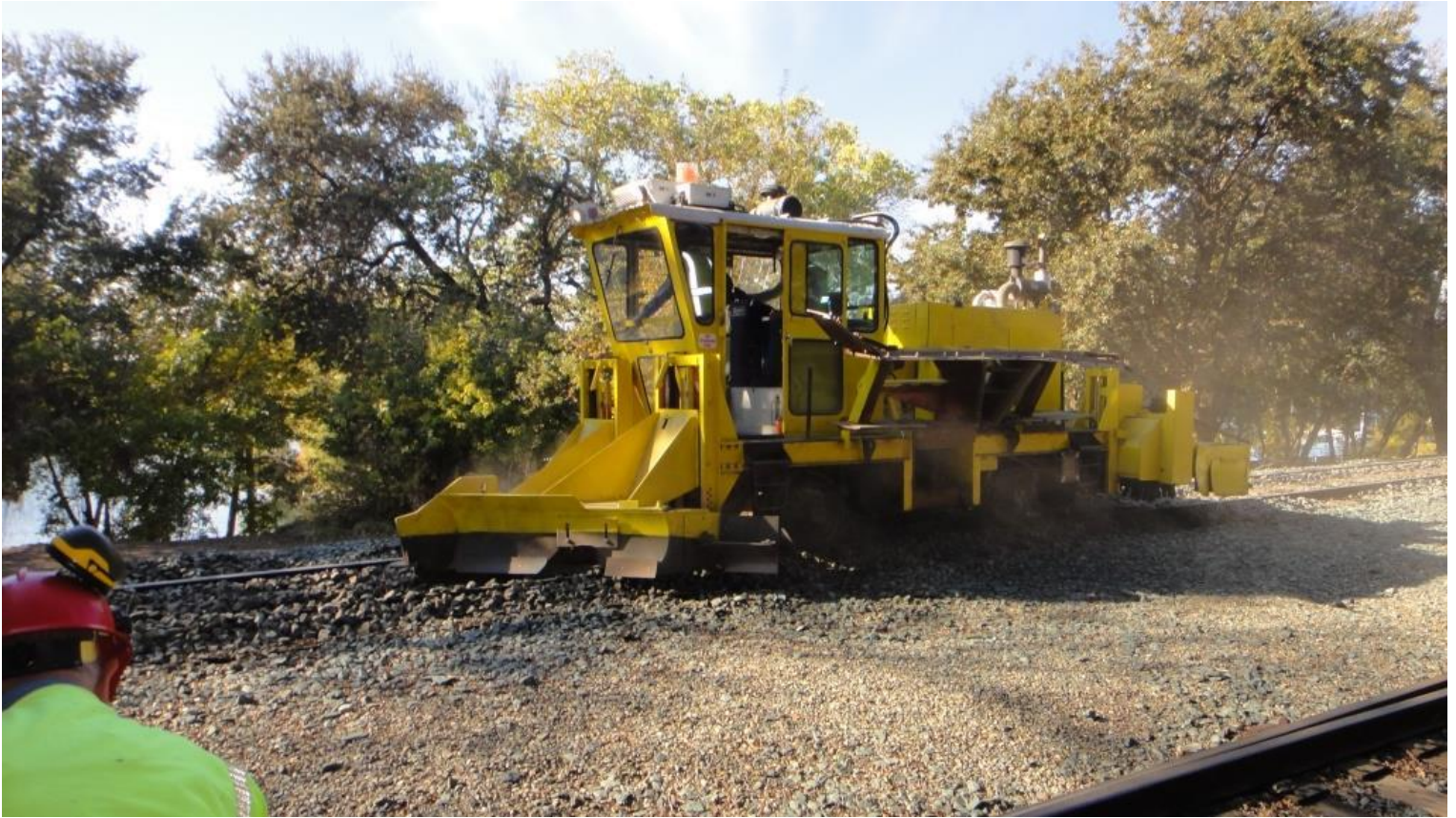
It's back to work and Chris N. takes a stab at operating the ballast regulator
